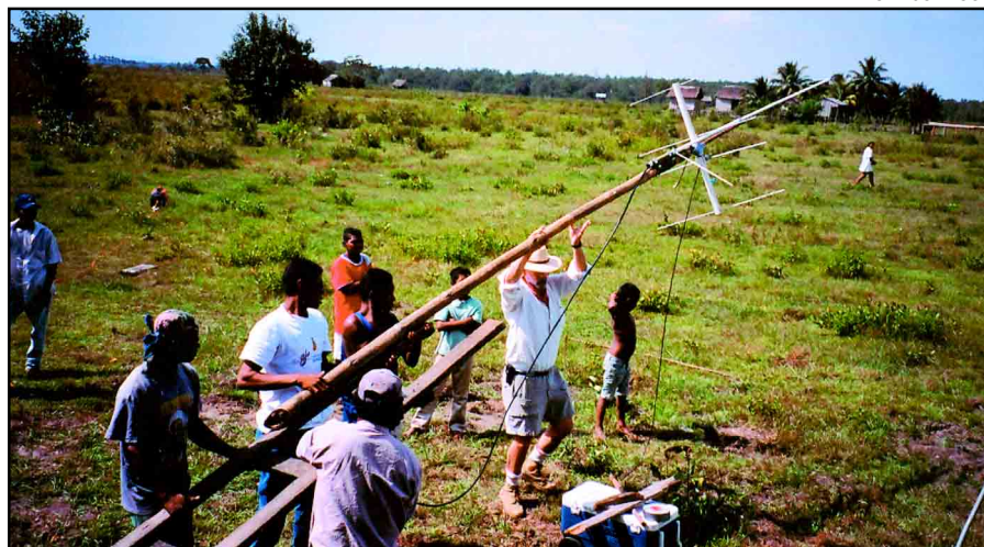
The author erects antenna mast for experimental 2 meter beam and HF Delta loop.
