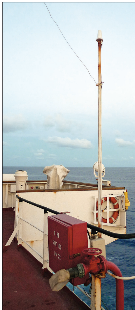
This is the end-fed sloper antenna located on the bridge deck, approximately 85 feet over the water. The remote tuner, located behind the fire station hose box, is mounted and grounded to the handrail.
